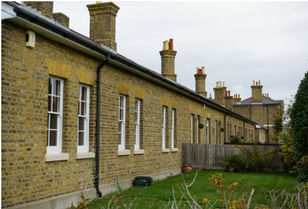
Row of NCO's quarters (No.30 Chapel Road and Nos.18-22 Hospital Road)
