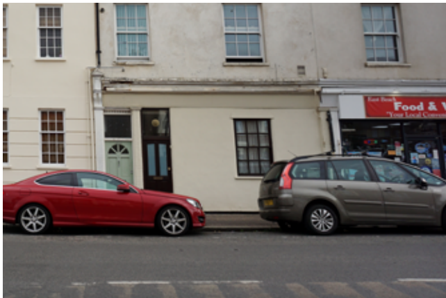
Domestic door and window added into former shop front
