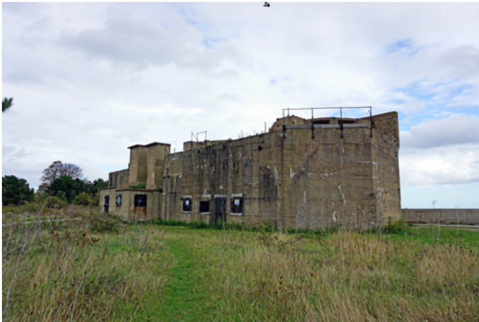
East elevation of the Heavy Quick Firing Battery
