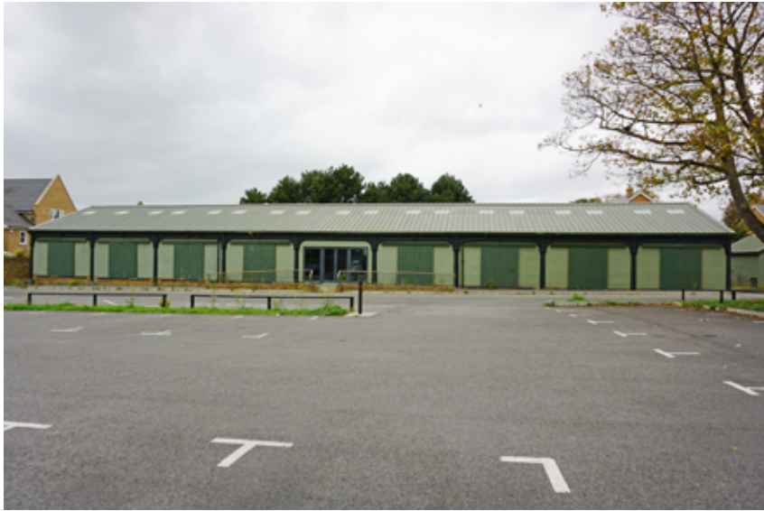
Carriage and Wagon Shed
