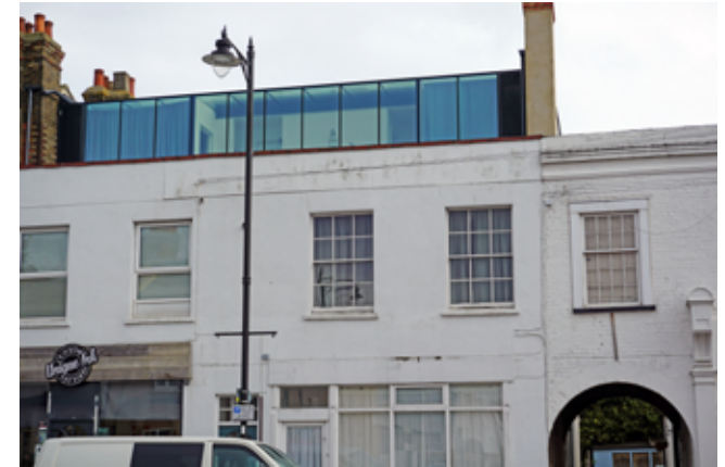
Out-of-keeping glazed rooftop extension, plus uPVC windows on buildings on the High Street
