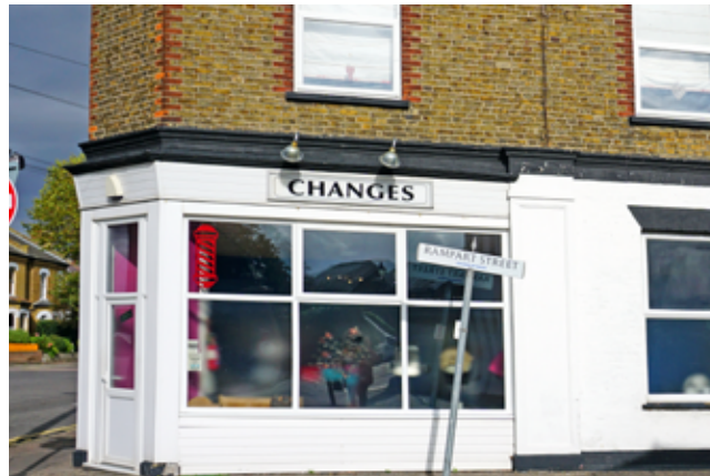
Inappropriate uPVC shop front
