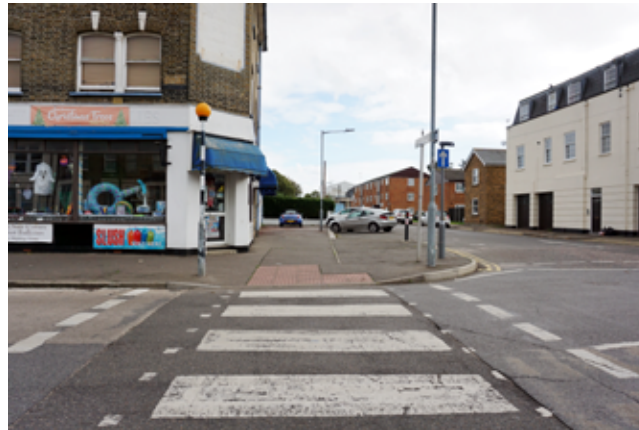
Utilitarian public realm features on the High Street, including Belisha beacon in need of replacing
