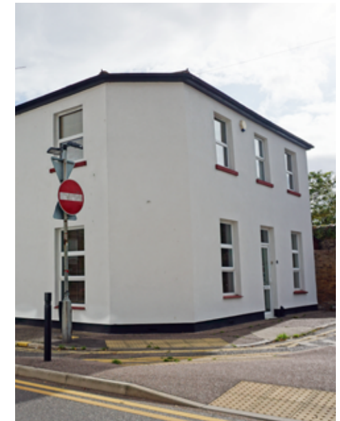
Appearance of No.2 High Street today, with door and shop window removed, render added over brickwork and timber sash windows replaced since the last Appraisal in 2004 with uPVC top hung units
