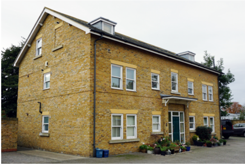
Flats to the rear of Horseshoe Crescent
